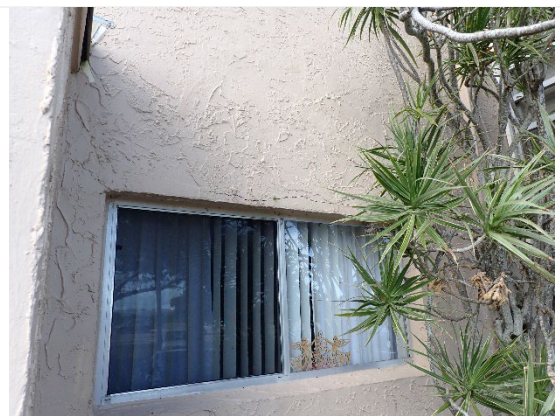
Photograph 10: Header Damage
