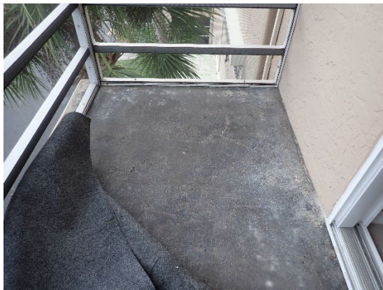
Photograph 5: Carpet on Balcony
